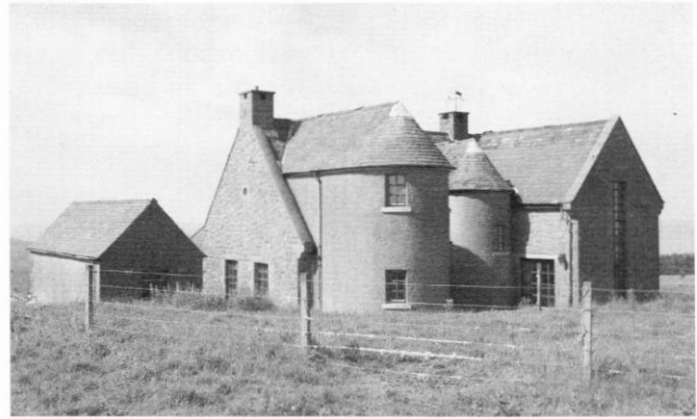
Rear of Crosslaw guardhouse after conversion. Photo by Gavin Saxby
